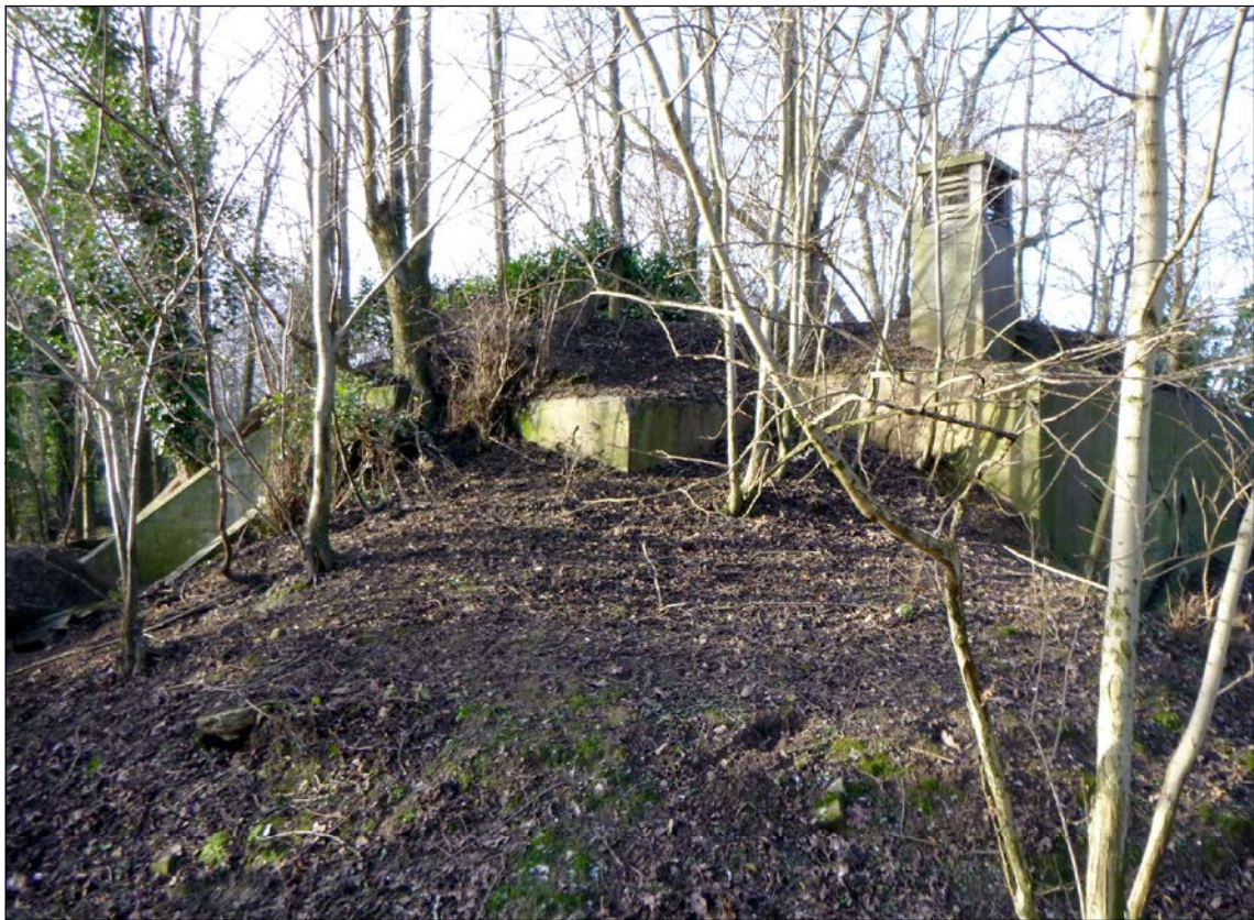
Plate 29) Chain Radar Building 2
