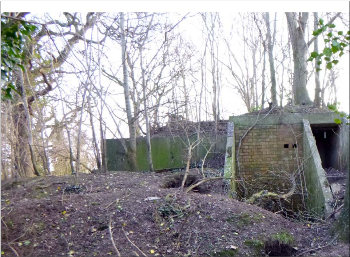
Plate 30) Chain Radar Building 2
